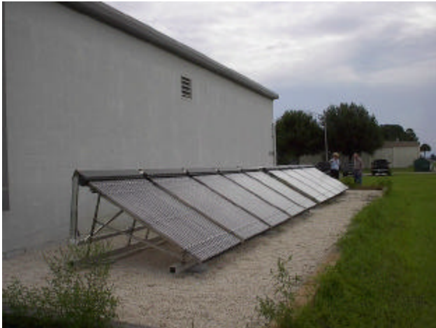
Figure 8: The Thermomax tubes at the Kennedy Space Station in Florida supplies 53,000 BTUH (200 + °F) to drive desiccant cooling units.
