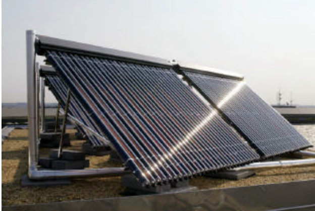
Figure 7: The Pentagon evacuated heat pipe solar system is the largest solar thermal system of its type in North America with a rated peak thermal output of 75.6 kW.
